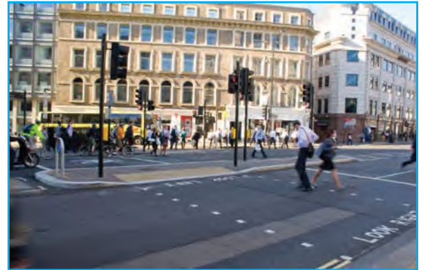
Staggered signalised crossing without guardrail
