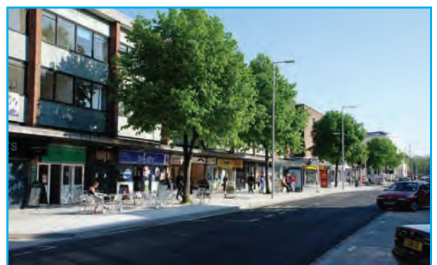
The London Road, Southampton scheme omits central line markings for part of its length.
