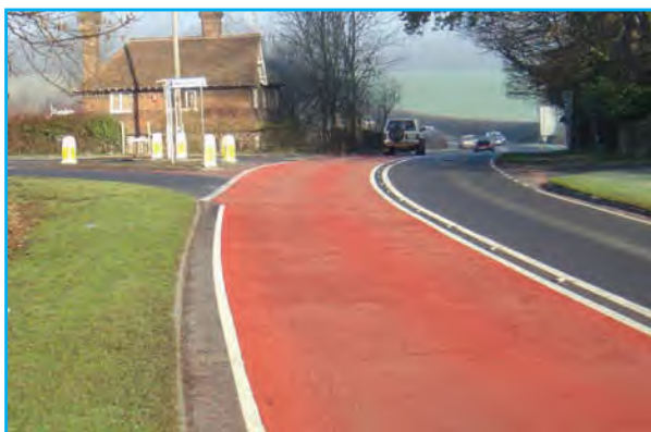
Excessive use of coloured surfacing can be visually intrusive
