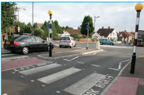
Zebra crossing close to mini-roundabout exit.
