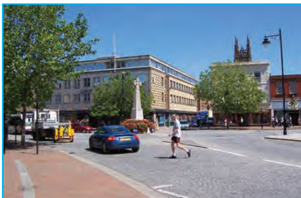
Roundabout in Taunton town centre with proceed left signs to Diagram 606 but no black and white chevrons to diagram 515. Note - cobbled surface is difficult for cyclists.
