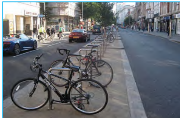
Cycle parking on central reservation, Kensington High Street. Generous spacing between the cycle racks enables pedestrians to cross between the parked cycles.
