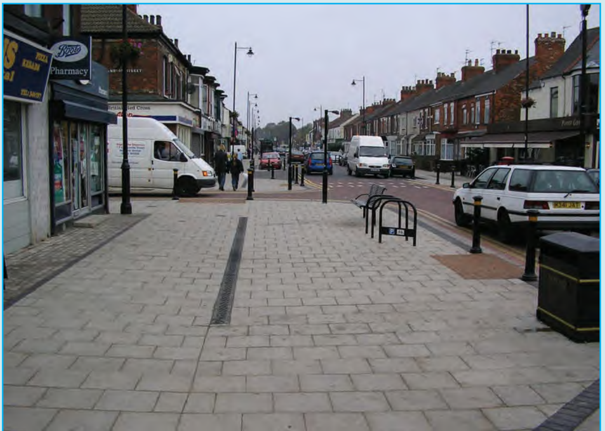
Footways widened significantly by narrowing carriageway
