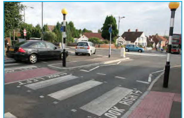
Zebra crossing located close to road junction.
