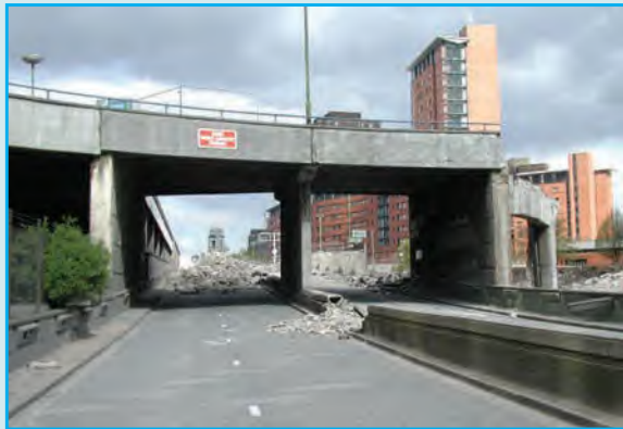
Breaking the Concrete Collar In Birmingham
