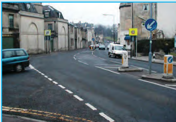
Julian Road Bath – Before and After
