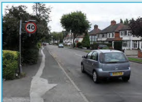
Single Lane, Frontage Access, On-Street Parking
