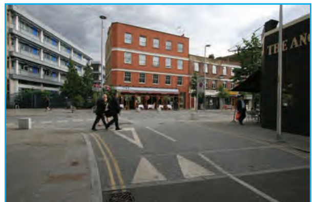
This junction has the Give Way marking (1003) and the approach triangle (1023) but no Give Way sign. It would have been possible to omit the approach triangle. Note also table to slow speeds and make pedestrian crossing easier.
